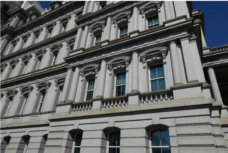
Photo 18. South elevation, view northwest.
