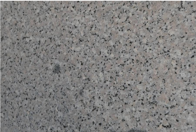
Photo 24. Detail view of substructure granite on east elevation.
