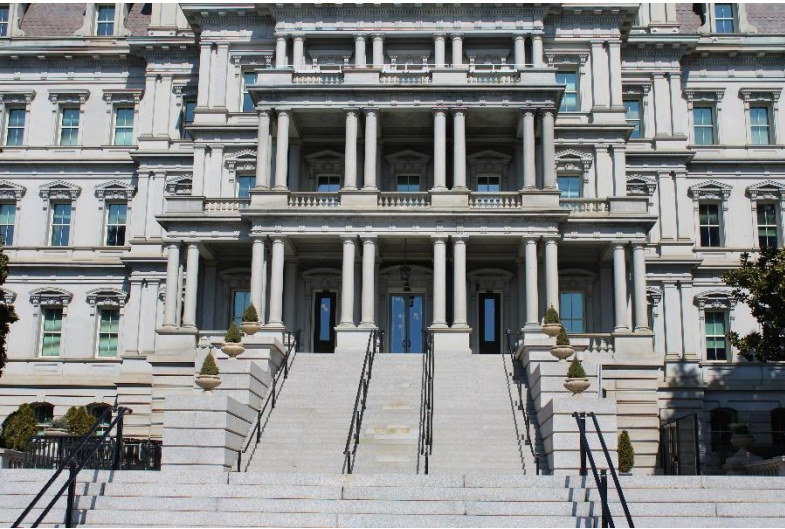
Photo 17. South elevation, view north.
