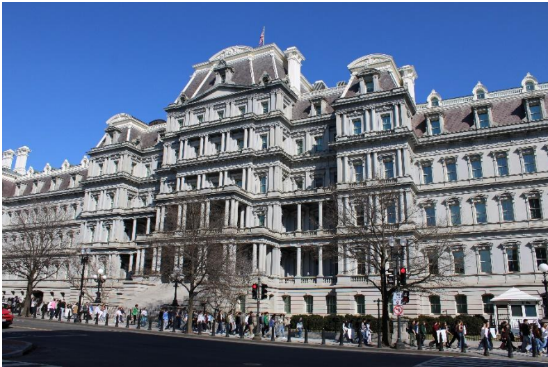
Photo 8. West elevation, view east.
