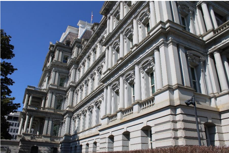
Photo 15. South elevation, view northwest.
