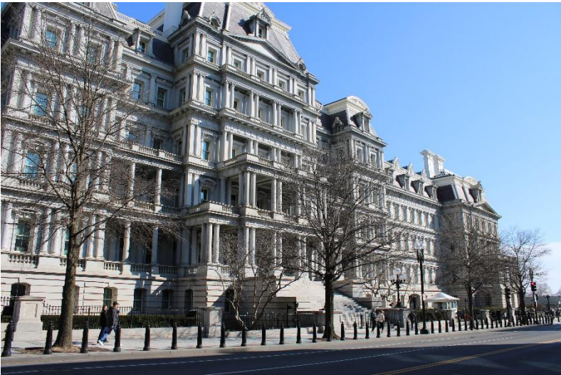
Photo 7. West elevation, view southeast.
