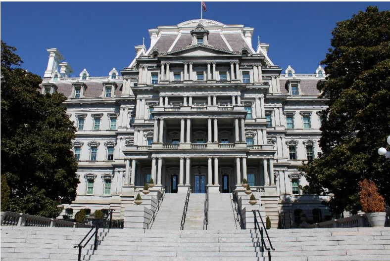
Photo 13. South elevation, view north.
