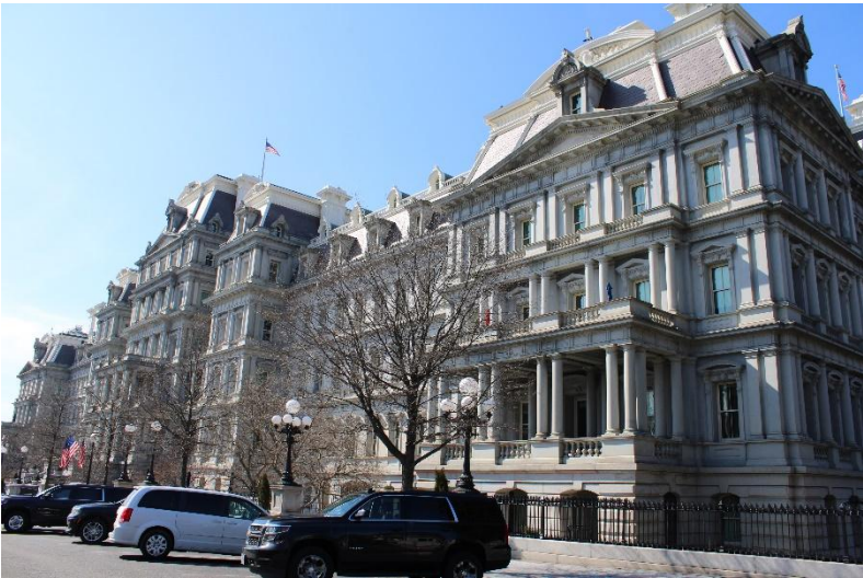
Photo 19. East elevation, view southwest.
