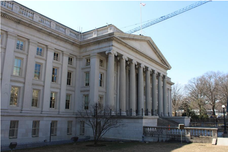
Photo 36. U.S. Treasury Building, north elevation, view southwest.
