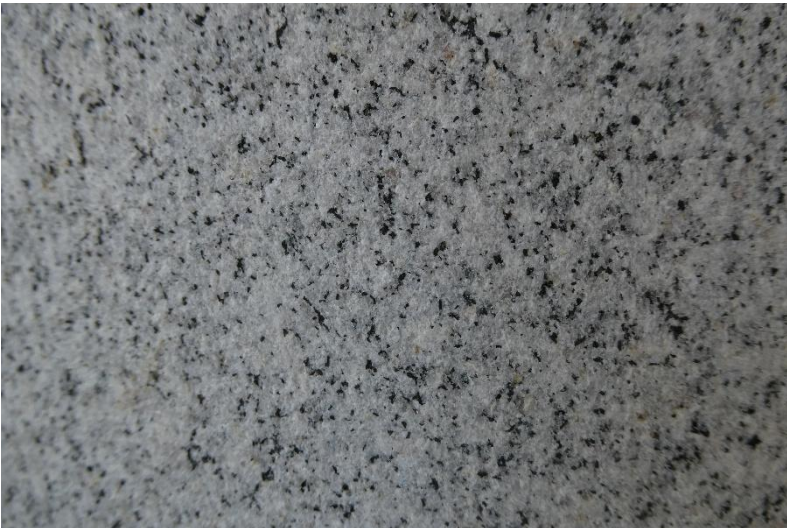
Photo 21. Detail view of superstructure granite on east elevation.
