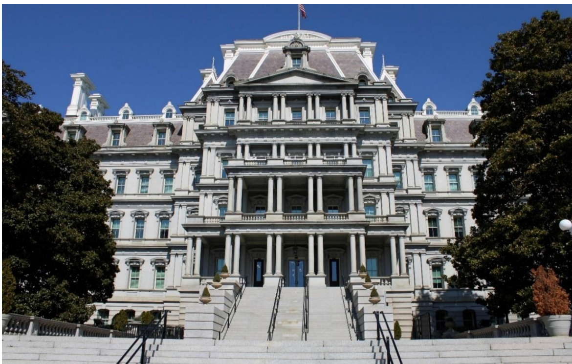
Figure 2. EEOB, south elevation, 2026.
