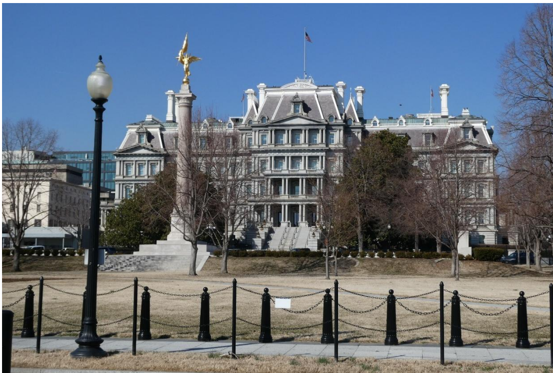
Figure 5: South elevation of the EEOB, view north, 2026.
