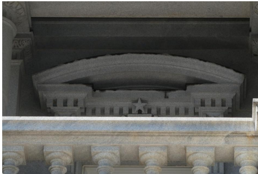
Figure 9: Gypsum salt accumulation in covered pavilion of EEOB, 2026.
