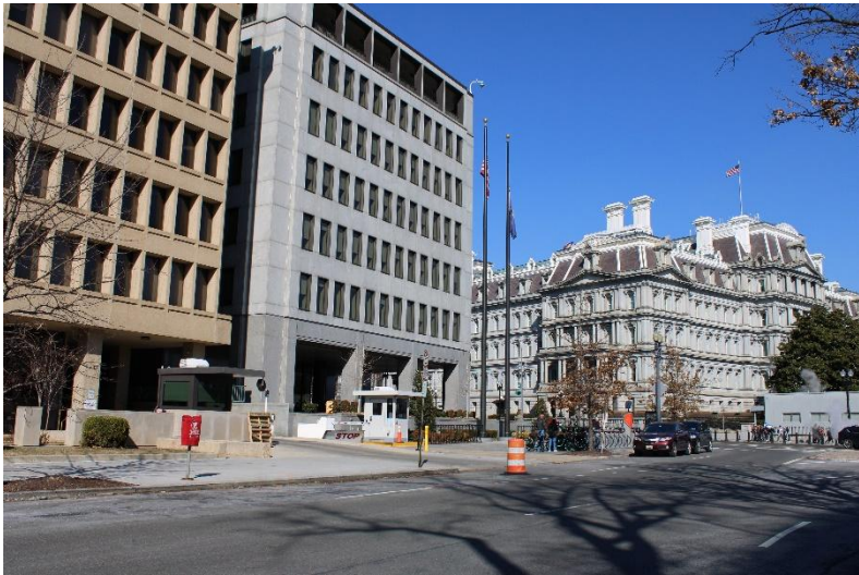
Photo 26. View northeast along New York Avenue, NW.
