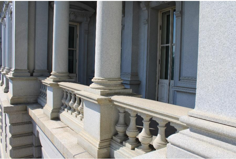
Photo 23. East elevation detail, view southwest.
