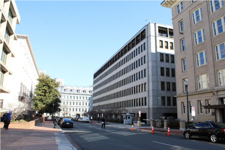
Photo 38. View southeast along F Street, showing the Civil Service Commission Building ( far right ) and EEOB ( center-background ).
