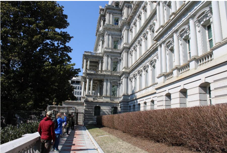
Photo 16. South elevation detail, view west.
