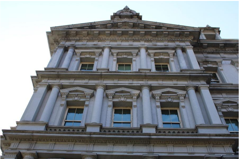
Photo 4. North elevation detail, view south.
