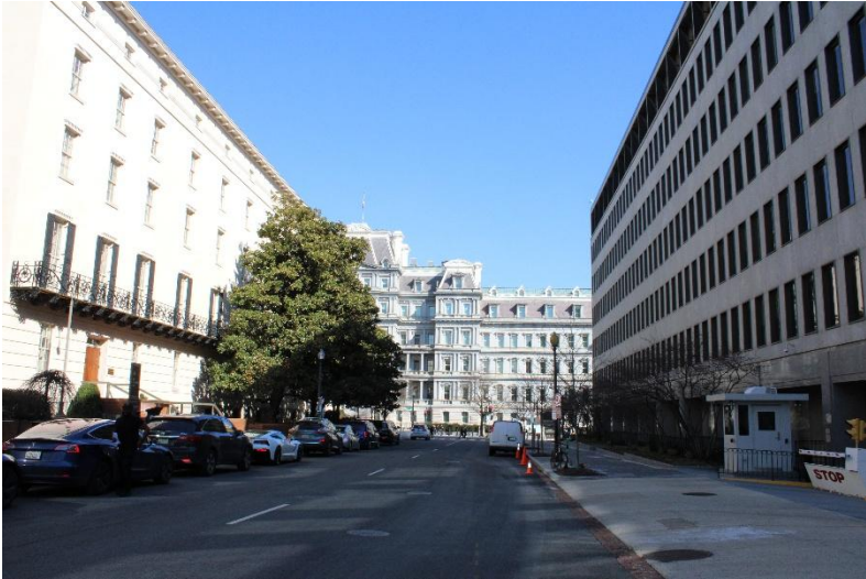
Photo 39. View east along F Street, showing the Winder Building ( left ) and the EEOB ( center ).
