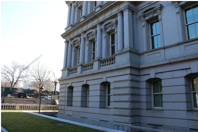
Photo 3. North elevation, view southeast.
