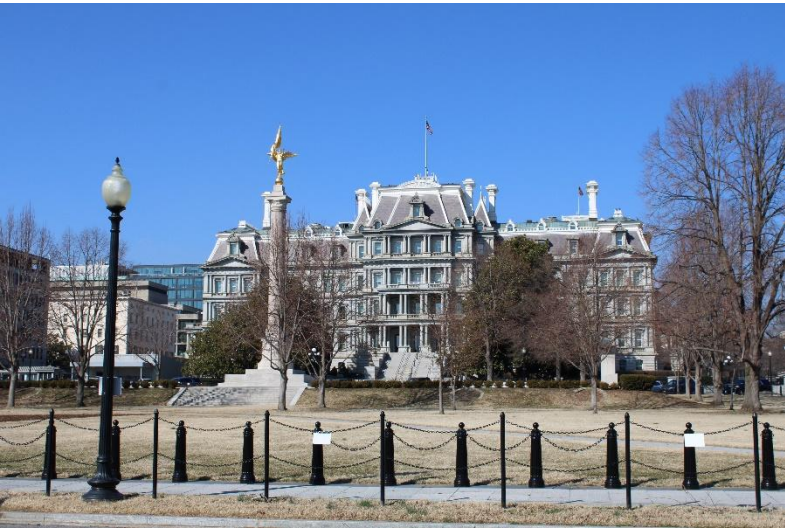
Photo 14. South elevation, view north.
