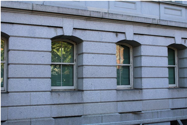
Photo 5. North elevation detail, view southwest.
