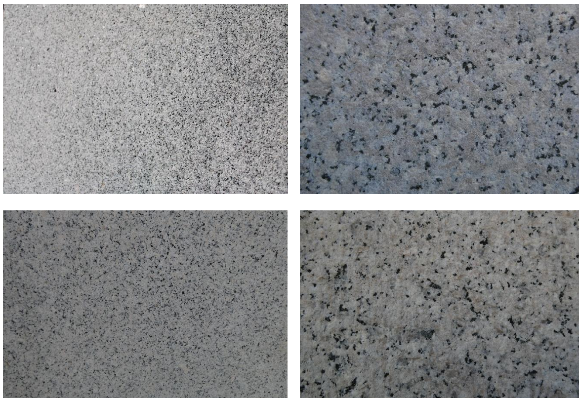
Figure 6: Detail views of granite from the superstructure of the EEOB ( top left ), the substructure of the EEOB ( top right ), the Treasury Building ( bottom left ), and the Old Post Office ( bottom right ).
