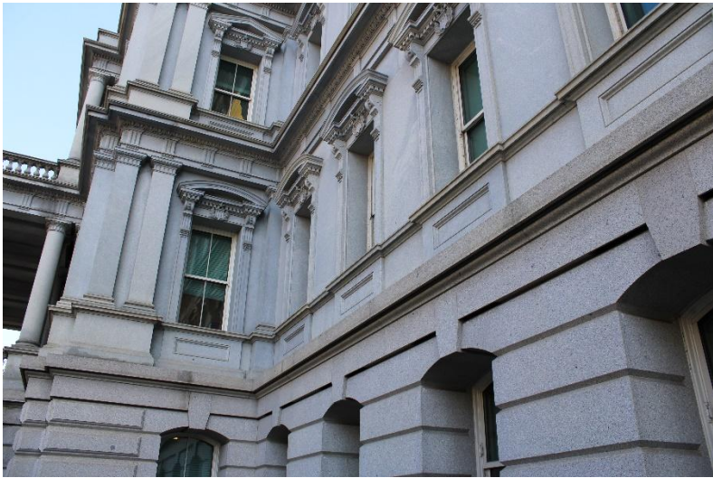
Photo 11. West elevation detail, showing subtle distinction between substructure and superstructure granite, view north.
