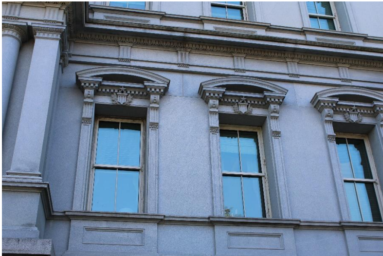
Photo 6. North elevation detail, view south.
