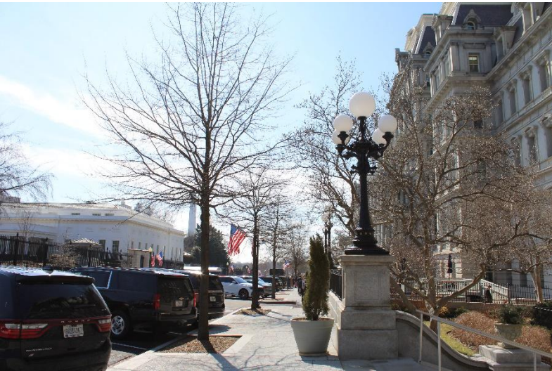
Photo 20. East elevation, view south.
